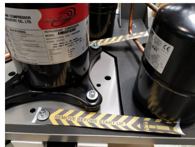
Figure 5.1 Removal of transport safety devices
